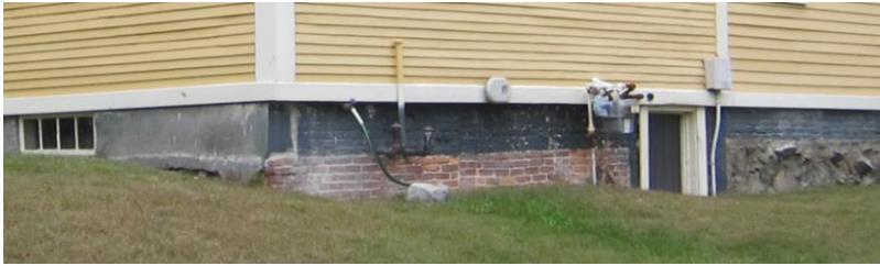
Mixture of brick, stone and granite foundation
