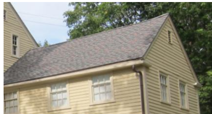
Asphalt shingle roof
