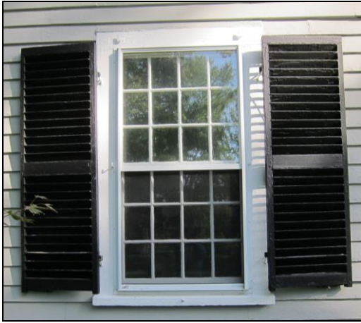
12/12 double hung sash with exterior storm
