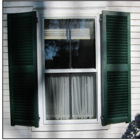
2/2 double hung sash with exterior storm
