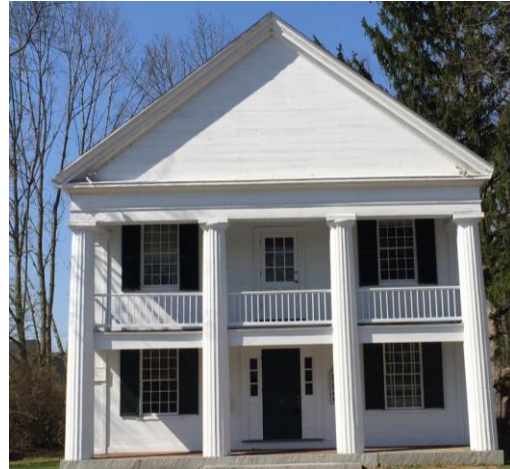
Wood flushboard siding in gable peak
