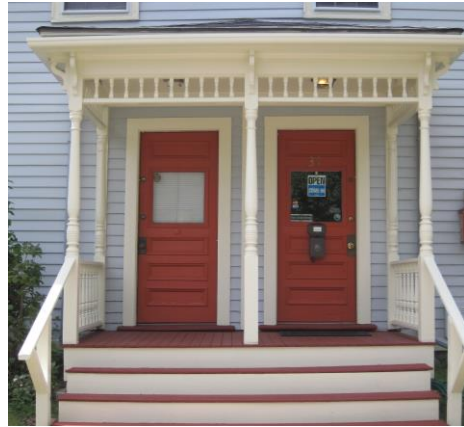
Paneled doors with square lights
