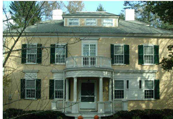
Colonial Revival hipped roof shallow dormer
