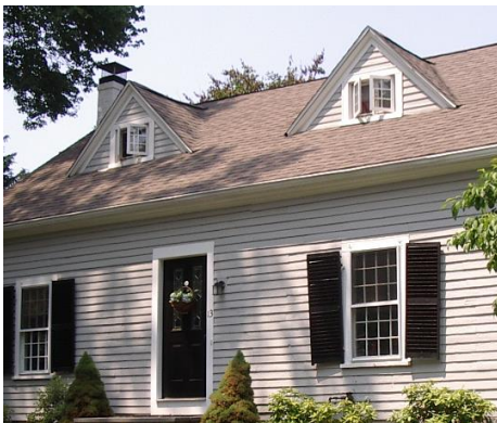
Small triangular dormers on main façade
