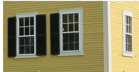
Plain window casing and corner board
