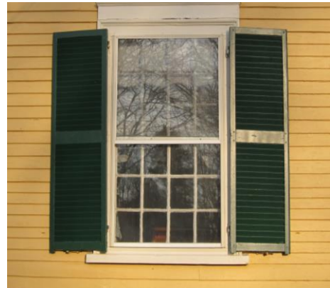
Closed shutters would cover sash
