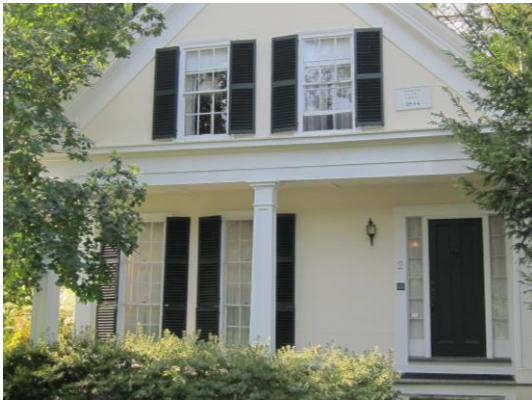
Full length wood louvered shutters flank windows
