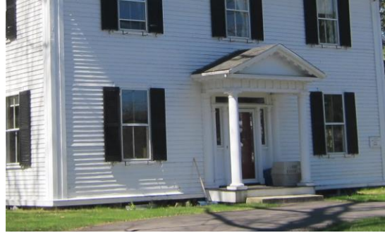
Colonial Revival entry porch
