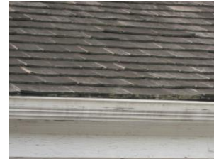
Wood shingle roof
