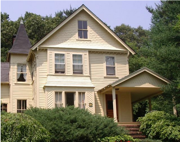
Patterned shingles and clapboards
