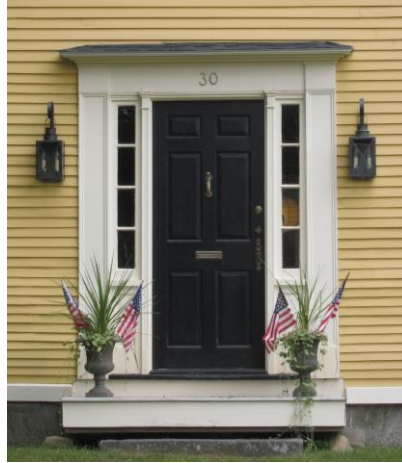
Six-paneled door with sidelights
