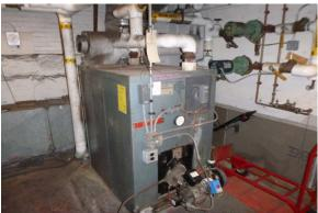
The existing oil-fired boiler serving the hot water system at the Town Library will be converted to natural gas.
