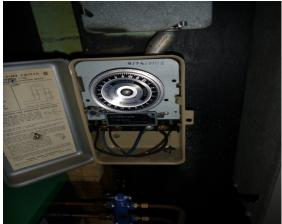
Time clock with no start/stop pins at Town Building will be replaced with Direct Digital Controls (DDC).
